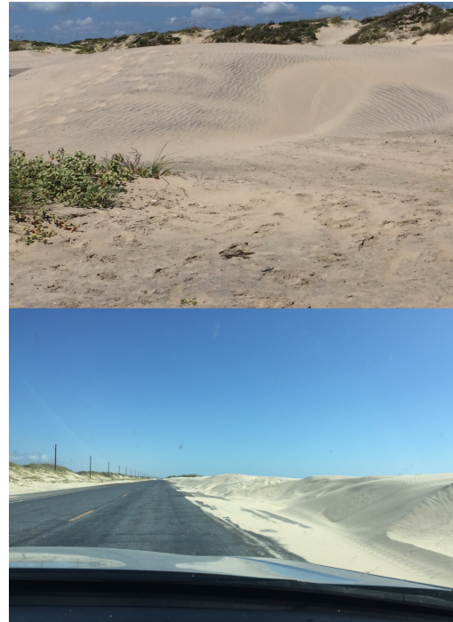
Figure 7. Barchan dune landform and sand deposition on Park Highway 100 at South Padre Island, Texas, 2017
