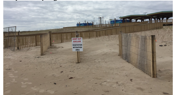
Figure 9. Recent integrated dune conservation program at Atwood Park, South Padre Island Texas, 2017: Revegetation, dune walkover, sand fences, designated parking and signage
